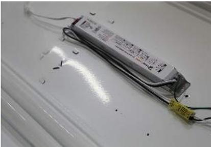
**STEP 5:** Replace the ballast cover and connect the wire harness so it is accessible.
