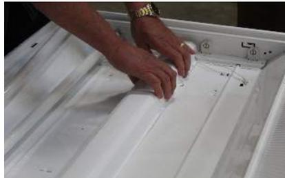
**STEP 6:** Clip Magnilumen's magnetic mounting brackets to the back of the LED boards.
