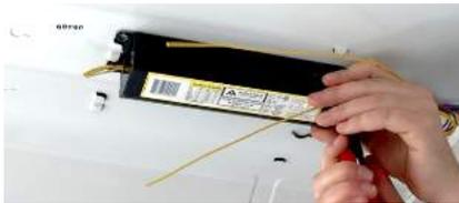
**STEP 2:** Place the Magnilumen magnetic driver into the fixture, and ground the driver.
