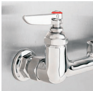
STEP 1 - Do NOT remove sink from wall. Locate connecting nuts.
